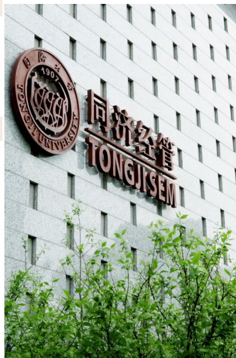
Tongji Building A
